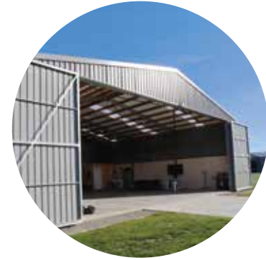
Hangars and umbrellas works
